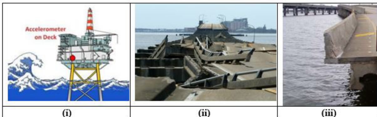
Figure 1: Wave impact on Ocean structures (i) Rogue waves hitting Draupner Platform (ii) Bridge damage during Hurricane Katrina (iii) Displacement of bridge deck
