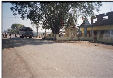
Reduction in Carriageway due to Roadside Encroachment
