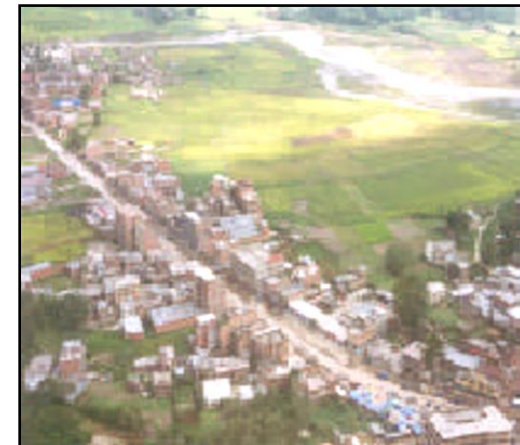
Aerial View of Ribbon Development Along Highway
