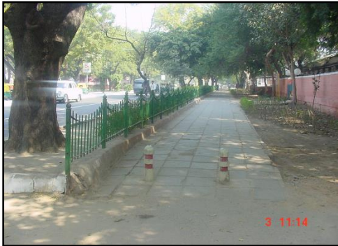
Pedestrian Segregated from the Traffic and the Barrier Provided to Restrict the Entry of Vehicles
