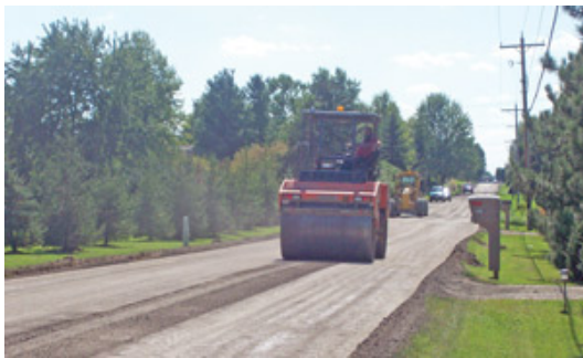
Figure 3. Compaction of FDR base
