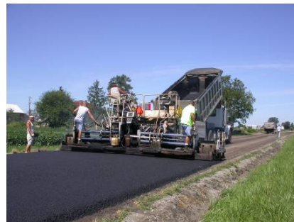
Figure 4. Resurfacing with hot mix asphalt
