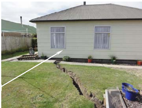
(b) Lateral spreading crack running through a residential property; (c) Lateral spread and slumping of the north stopbank of the Kaiapoi River; note the huge piles of cleaned up sand obstructing the view of the houses
