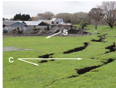
(b) Lateral spreading crack running through a residential property; (c) Lateral spread and slumping of the north stopbank of the Kaiapoi River; note the huge piles of cleaned up sand obstructing the view of the houses
