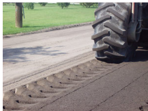
Figure 2. Blending fly ash with pulverized base
