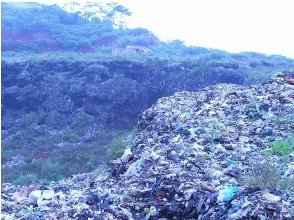
Photo 1 Top scarp of failed landfill
